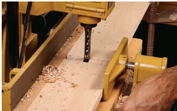
Mortises first. Mark the upper and lower stretchers for the location of the vertical drawer dividers, and then cut these through-mortises with a hollow-chisel mortiser, using a backer board to prevent blowout.
